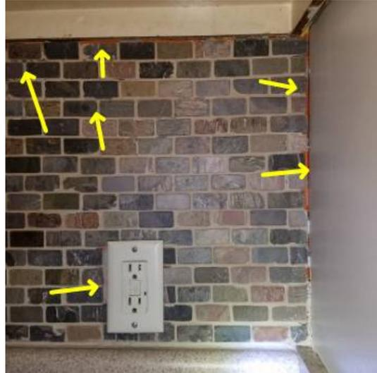
Figure 2.4 DEFECT Grout/tile work incomplete. Consult masonry contractor for work completion.
