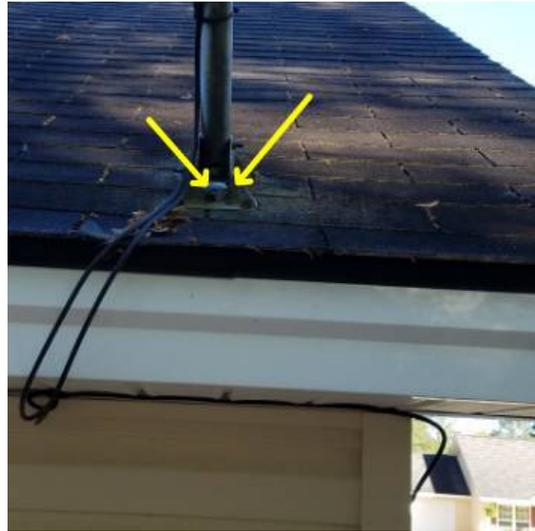
Figure 1.2 DEFECT Possible moisture intrusion point. No sealing measures taken in mounting of satellite dish. Consult roofing contractor for repair.
