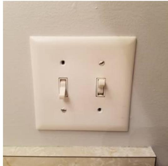
Figure 2.2 DEFECT Screws missing in switch plate in master bath.
