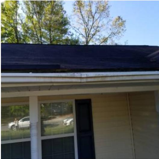
Figure 1.1 DEFECT Gutter sagging from apparent debris accumulation.
