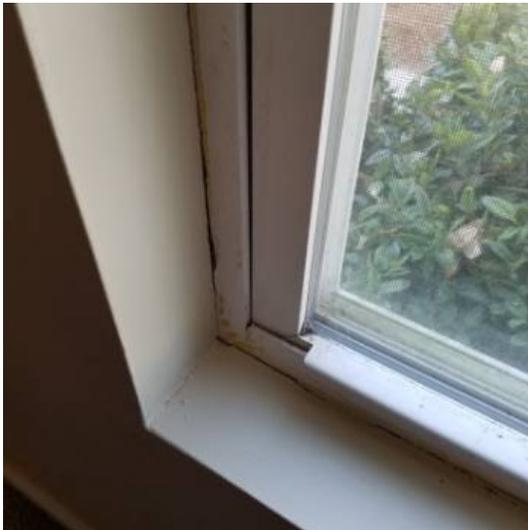
Figure 2.1 DEFECT Caulking broken around window.
