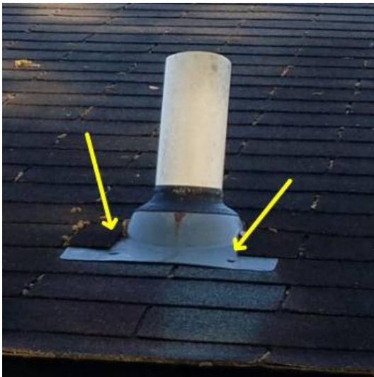
Figure 1.3 DEFECT Nails in flashing exposed. Possible water intrusion point. Condition on all vent pipes on roof. Consult roofing contractor for repair.
