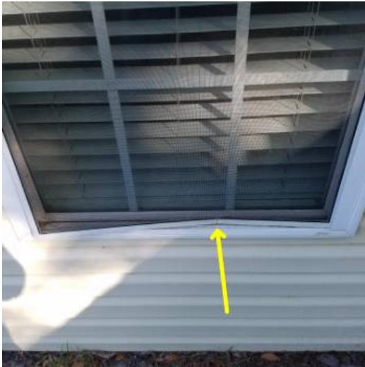
Figure 1.5 DEFECT Damaged Screen.
