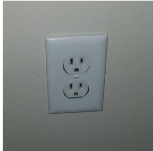
Figure 2.8 DEFECT Guest bedroom outlet not properly secured in guest bedroom facing front side of house. Consult Electrician for repair estimates.
