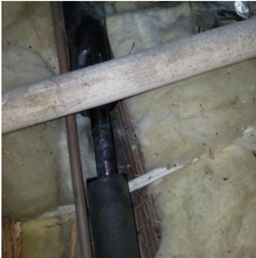
Figure 2.3.1 Insulation on Low Pressure refrigerant line in attic causing moisture in attic to condense into a liquid and falling on Ceiling joists. This can over time cause a mold issue as well as drywall damage if not corrected. Recommend Contacting HVAC Service Technician for repairs. if not corrected.
