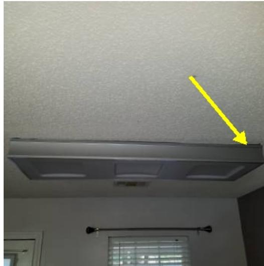
Figure 2.9 Light fixture apparently sagging posing possibility of part or all of the fixture falling. Consult with electrician to have re-mounted properly.
