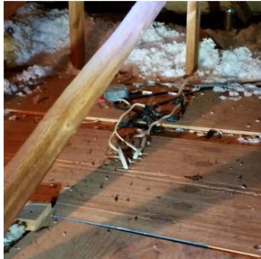
Figure 2.3.2 DEFECT Improper joining of Electrical conductors in attic. Recommend Contact qualified electrical service technician for assessment and repair.
