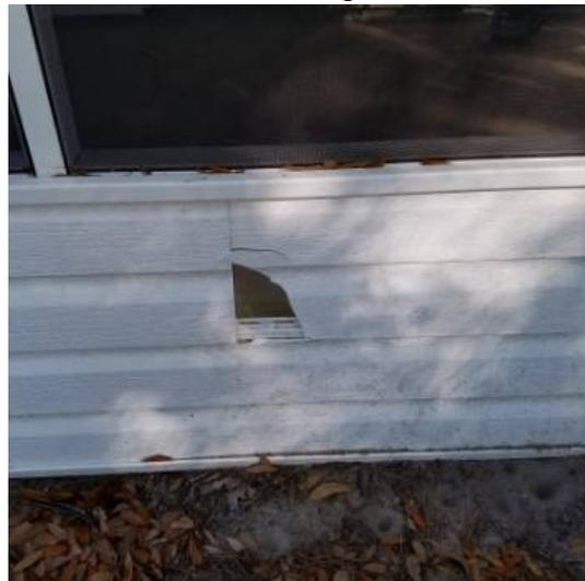
Figure 1.4 DEFECT Broken siding on rear of house.
