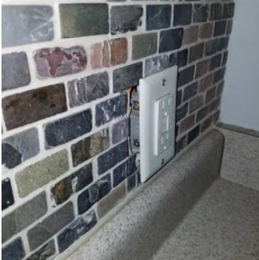
Figure 2.3 DEFECT Outlet/plate not secured to wall. Consult Electrician for repairs. Loosely mounted receptacles can move side to side causing ground fault.
