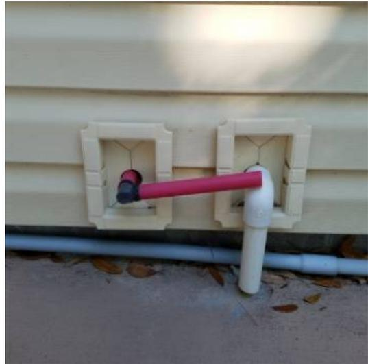
Figure 1.6 DEFECT Drain pipe not running downhill. Standing water left in line could create clog and cause drain to malfunction. Consult plumbing contractor for issue correction.
