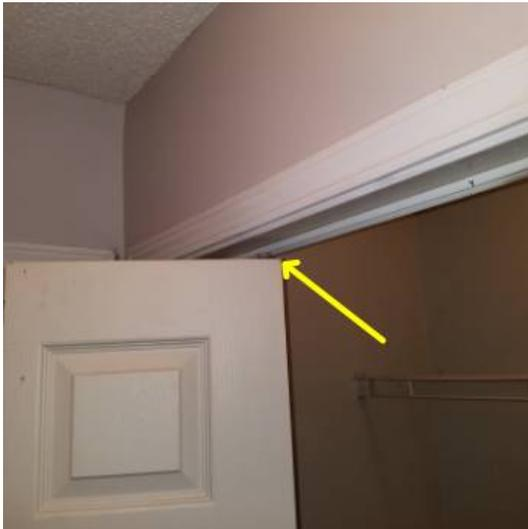
Figure 2.5 DEFECT Bifold doors not in track.
